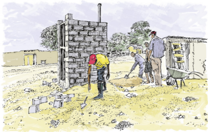
Figure 7. A VIP latrine under construction
