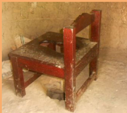
Lower cost wooden toilet seat, moveable so others can remove it and squat. Credit: WaterAid/WEDA.
