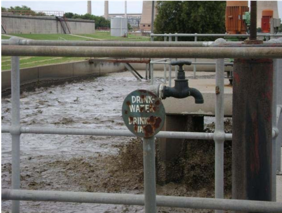
Fig. 40: Potable water tap, labelled but in very vulnerable position.
