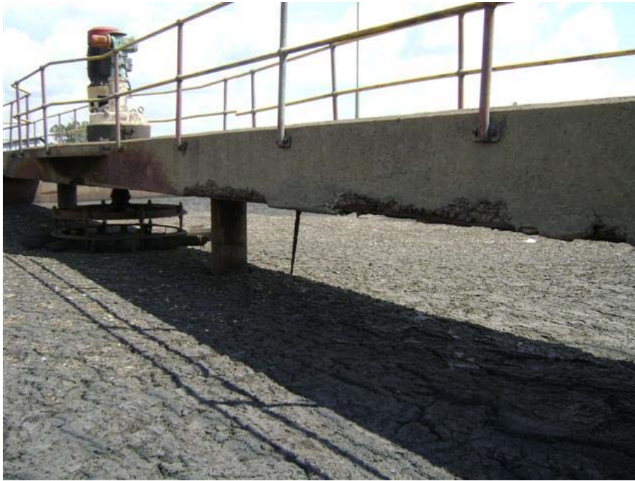
Fig. 71: Poor condition of BNR zone 2 shows septicity attack on bridge.
