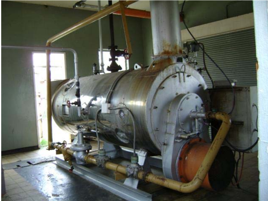
Fig. 10: Boiler out of use due to lack of gas.
