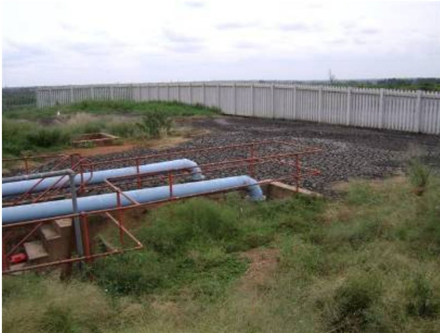
Fig. 30: Sludge overflows from holding dam.
