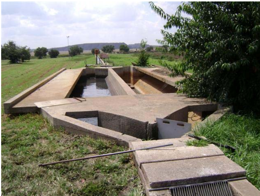
Fig. 68: Disused parallel grit removal channels.
