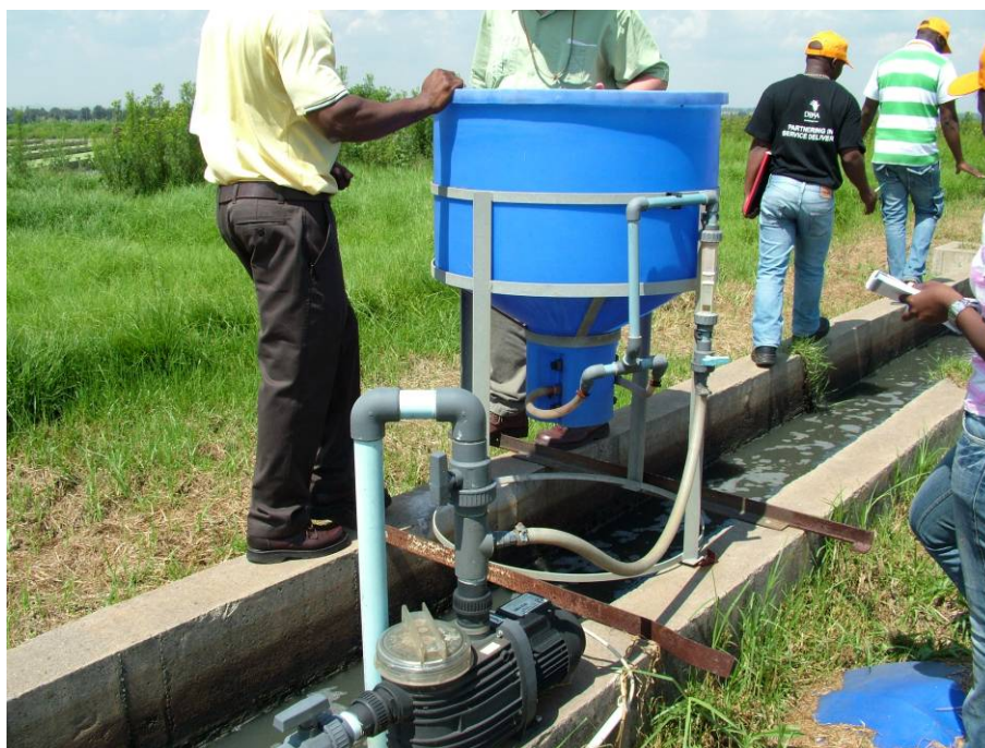
Fig. 76: Temporary Fix Chlorination unit, fixed but not functioning.
