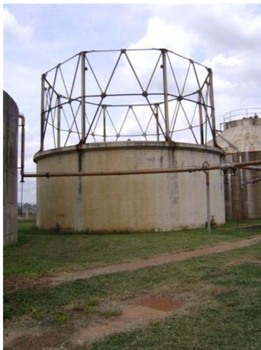
Fig. 9: Empty gas holder east works
