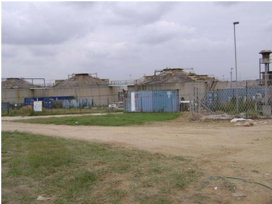
Fig. 46: Bank of 6 digesters, some in need of refurbishment.
