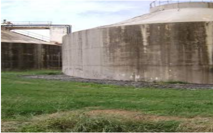
Fig.16: West works leaking digesters
