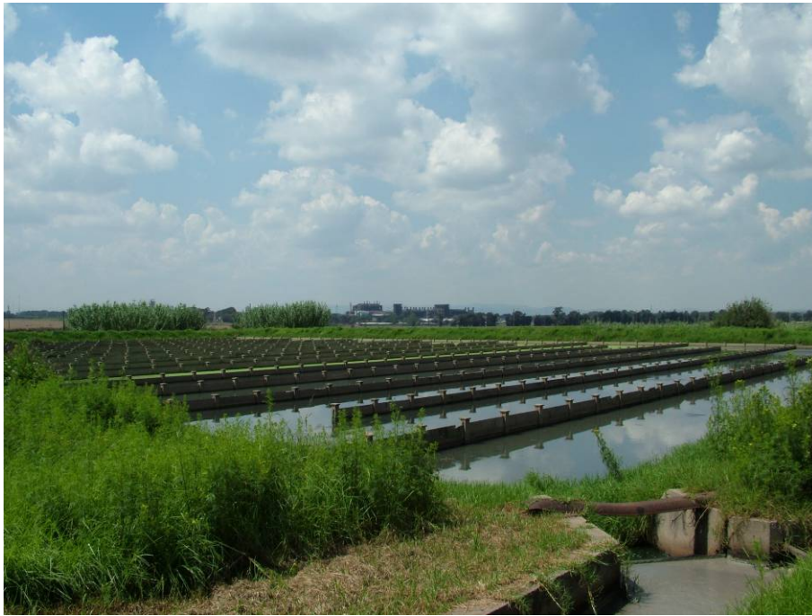
Fig. 77:Lagoon and contact tank, full of sludge and being bypassed.
