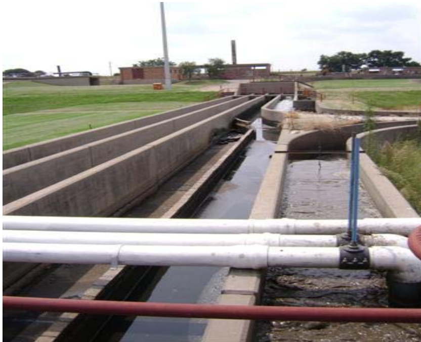
Fig.23: Above ground RAS pipelines feeding back to BNRs
