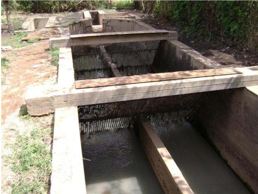
Fig. 61: Inlet screens channels with no fall protection provided.
