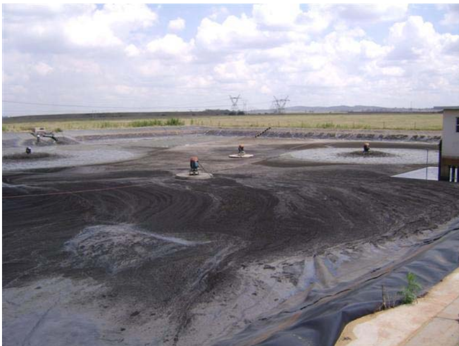
Fig. 66: New aerated balance pond with highly septic contents, showing aerators out of use
