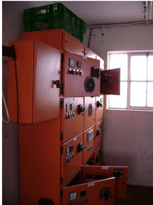
Fig. 85: Transfer ps with panel doors open, posing high risk of electric shock.
