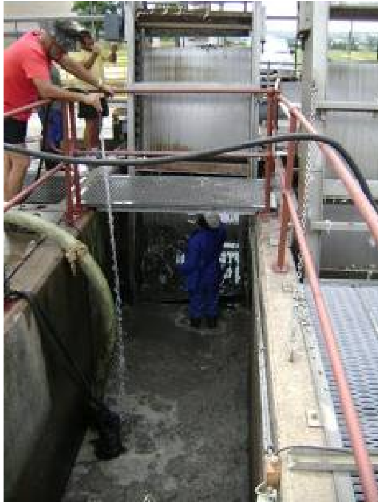
Fig 1: Mechanical Screen out of use and under repair. Also shows limited ppe
