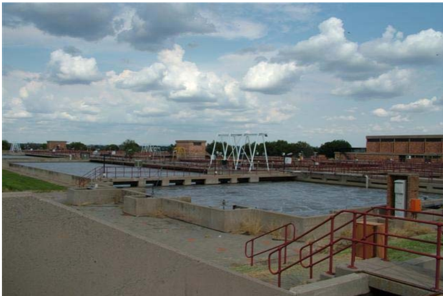
Fig. 19: BNR Reactors
