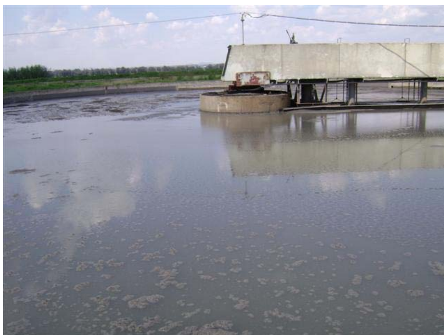
Fig. 75: FST Surface showing grey-black poor quality contents.
