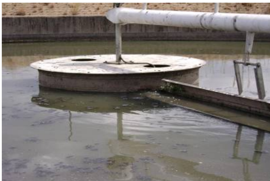
Fig. 6 Humus tanks overloaded
