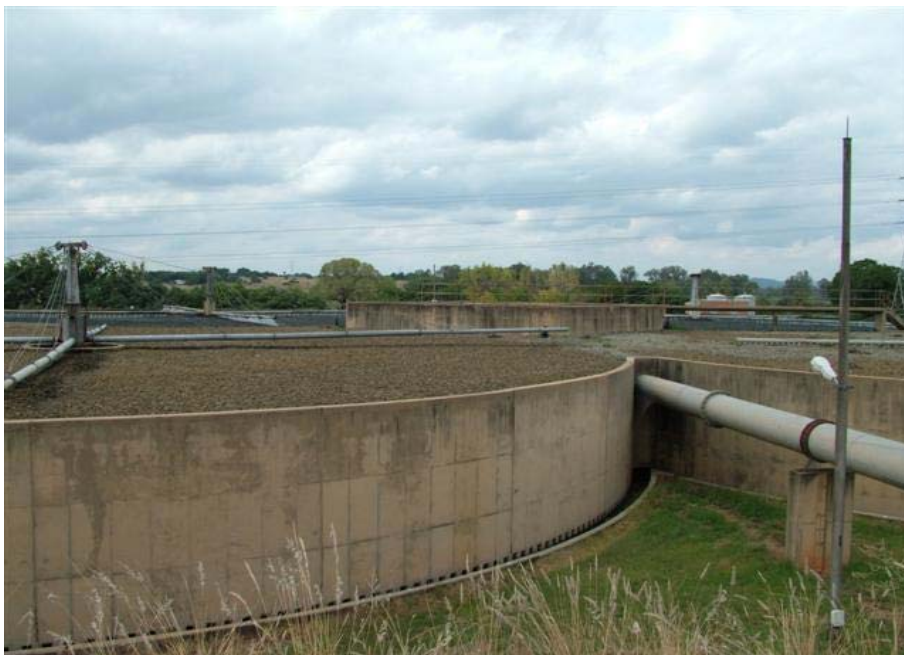
Fig 5: East works filters out of use due to mechanical issues.
