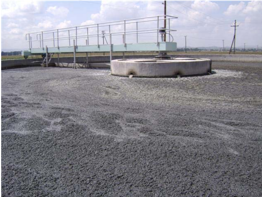
Fig. 65: New PST heavily overloaded, with thick scum of solids on surface.
