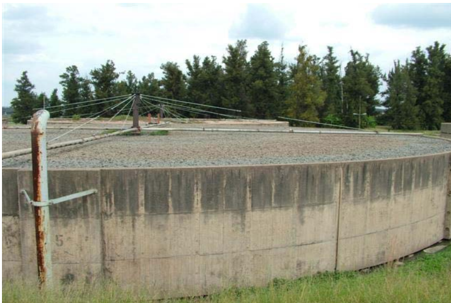
Fig.14: Biofilters totally out of use, mechanical plant missing
