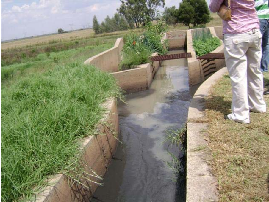
Fig. 67: Joining channel for flows from both inlet works.
