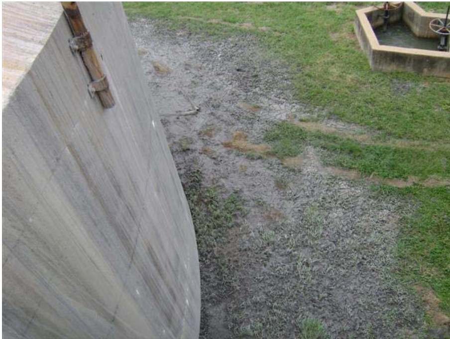
Fig. 8: Leaking digesters east works
