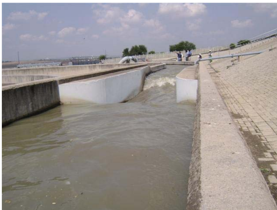
Fig. 44: Inlet channel very close to overflowing
