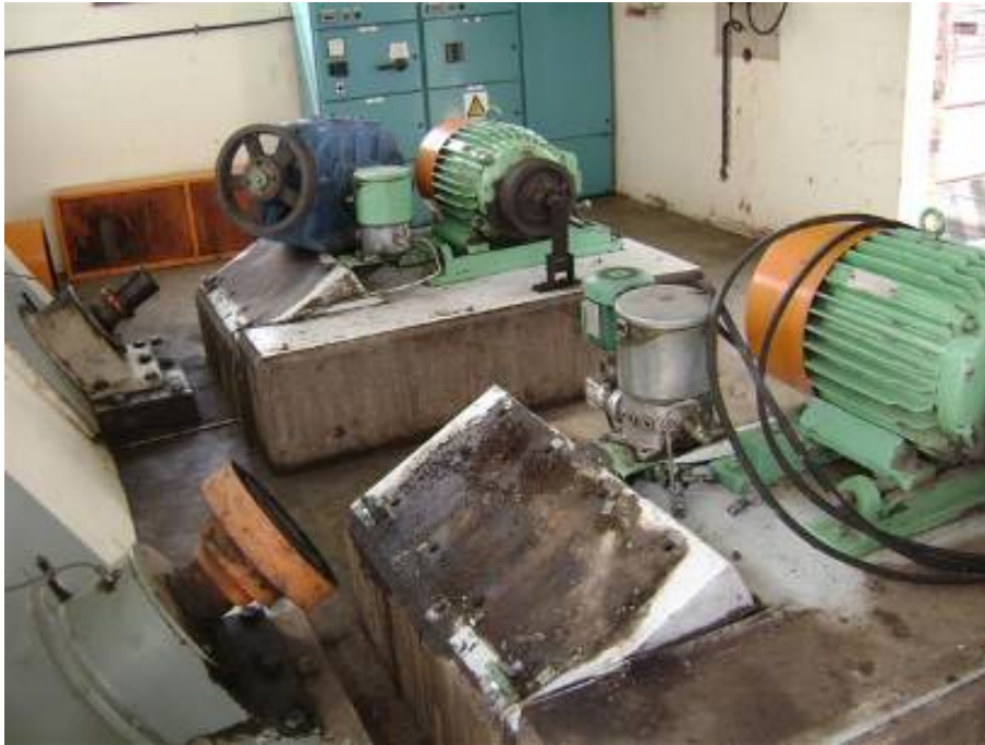
Fig.22: RAS screws taken out of action, pumps partially dismantled.
