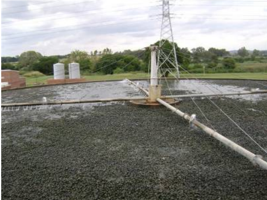
Fig. 4: East works biofilters ponding due to overloading
