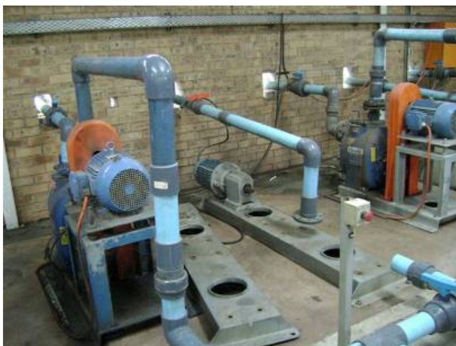
Fig. 35: Redundant polymer dosing equipment.
