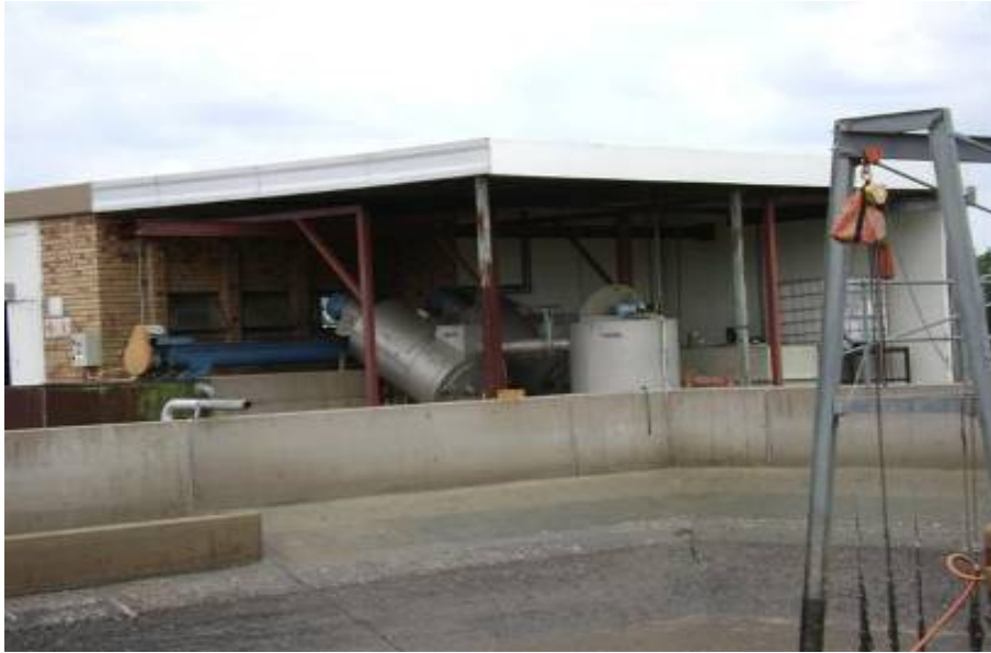
Fig. 26: Drum thickeners not being used.
