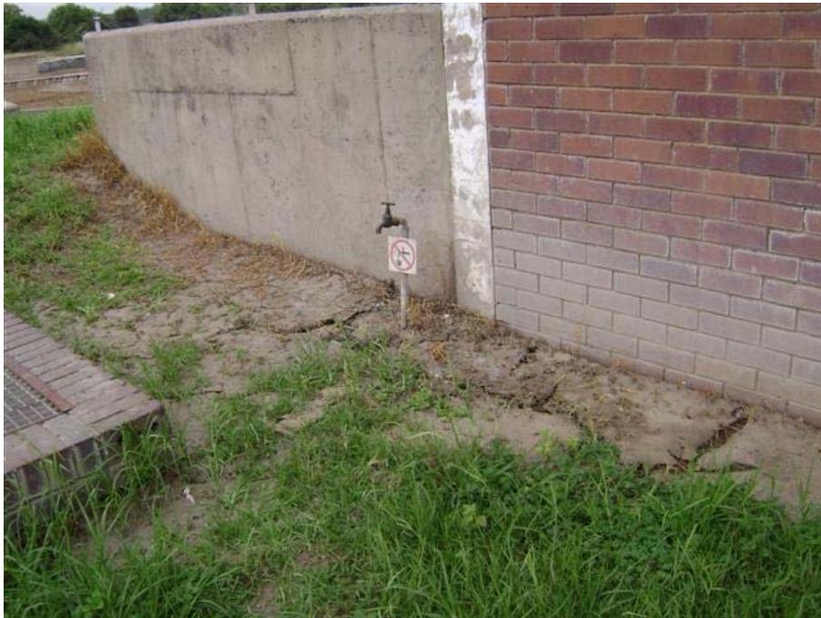
Fig. 24: Overflows from sludge transfer ps, around water (non potable) tap
