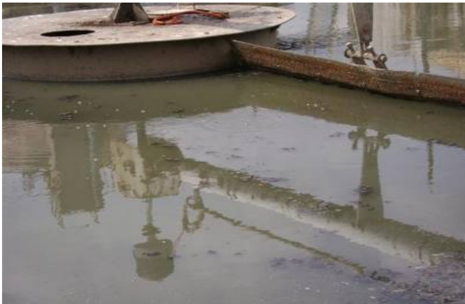
Fig.3: East works PST short-circuiting
