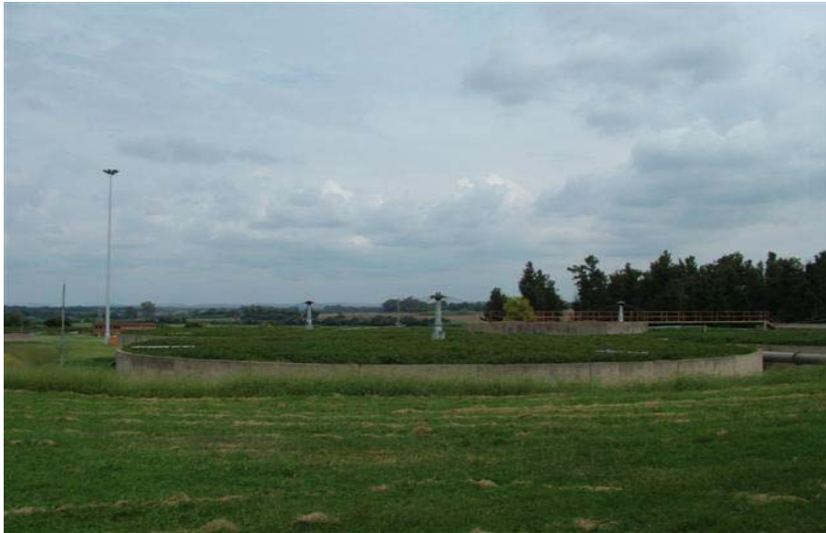
Fig. 15: Biofilters out of action due to mechanical issues, excessive vegetative growth.
