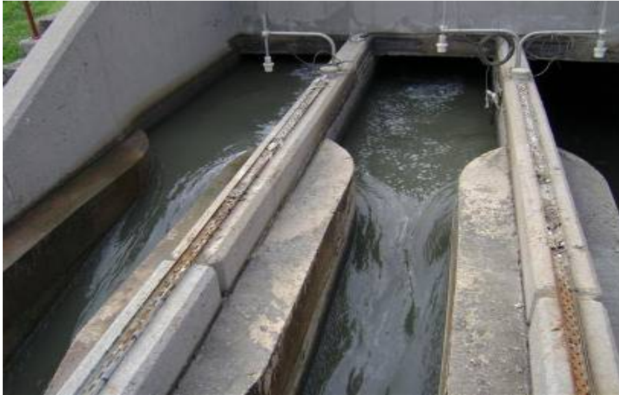
Fig. 18: Flooded inlet flumes
