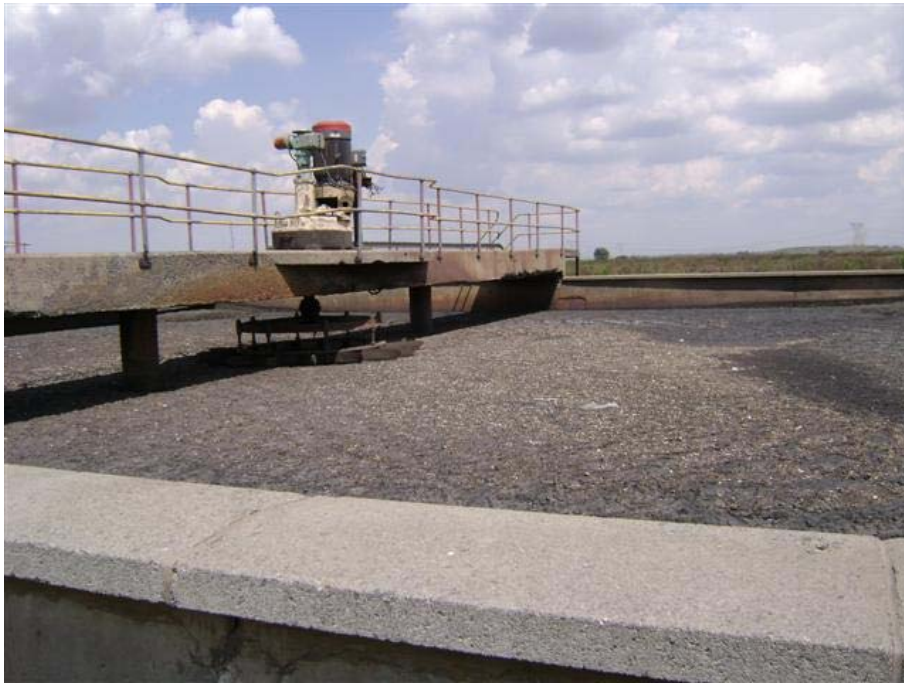
Fig. 73: BNR Zone 2 aerator out of action and heavy crust forming.
