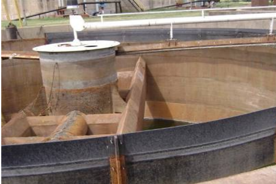
Fig.2 East Works PSTs out of use – mechanical failures
