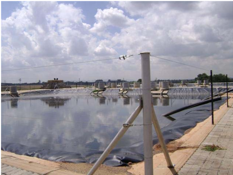
Fig. 78: New sludge digester, open topped.
