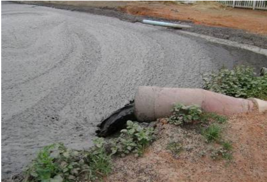
Fig. 28: Sludge dam inlet flows, shows close proximity of inlet pipes to banking.
