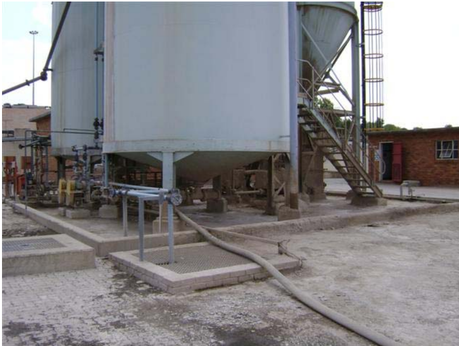
Fig. 51: Spillages around lime dosing plant not cleaned-up.
