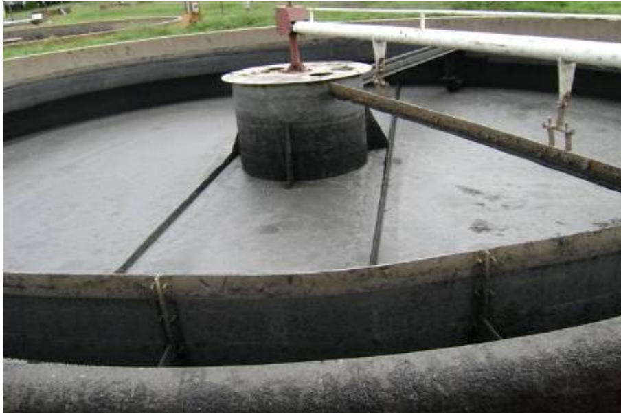
Fig. 13: PSTs being used to re-settle sludge from north works
