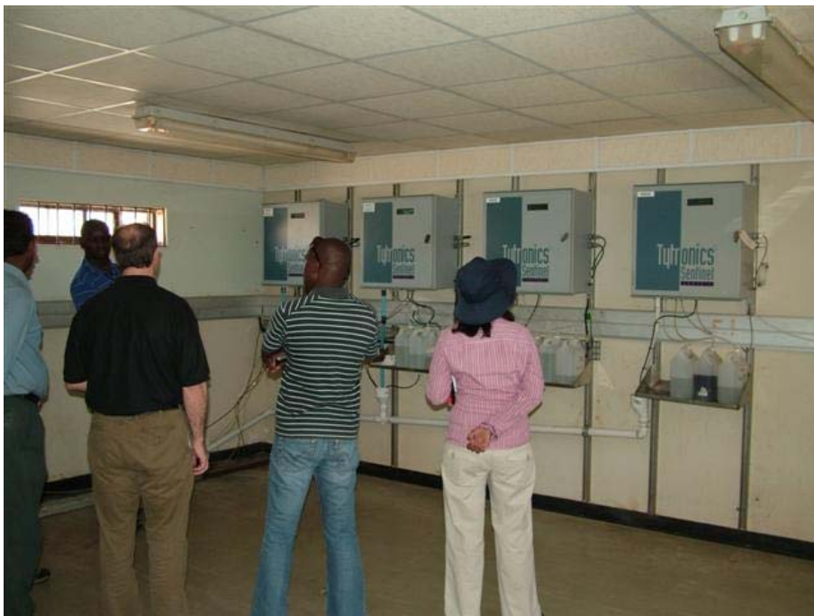
Fig. 52: Auto analysers monitoring various fe components.
