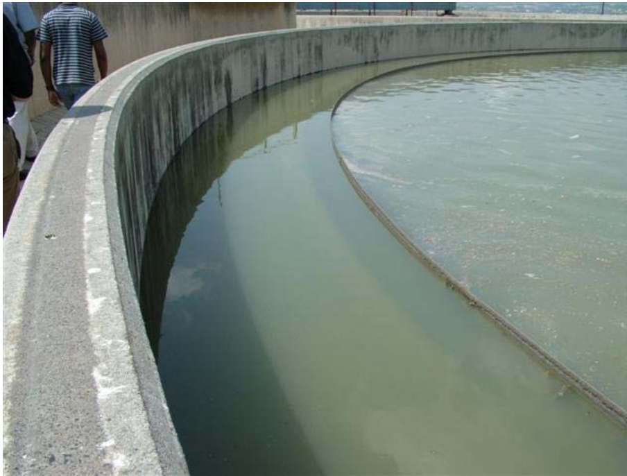
Fig. 45: PST Launder channel flooded due to hydraulic overloading
