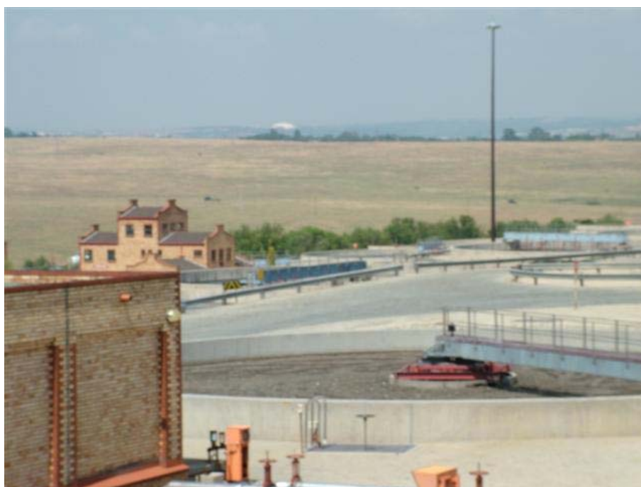
Fig. 54: PST out of action, showing crust formation, awaiting repairs.
