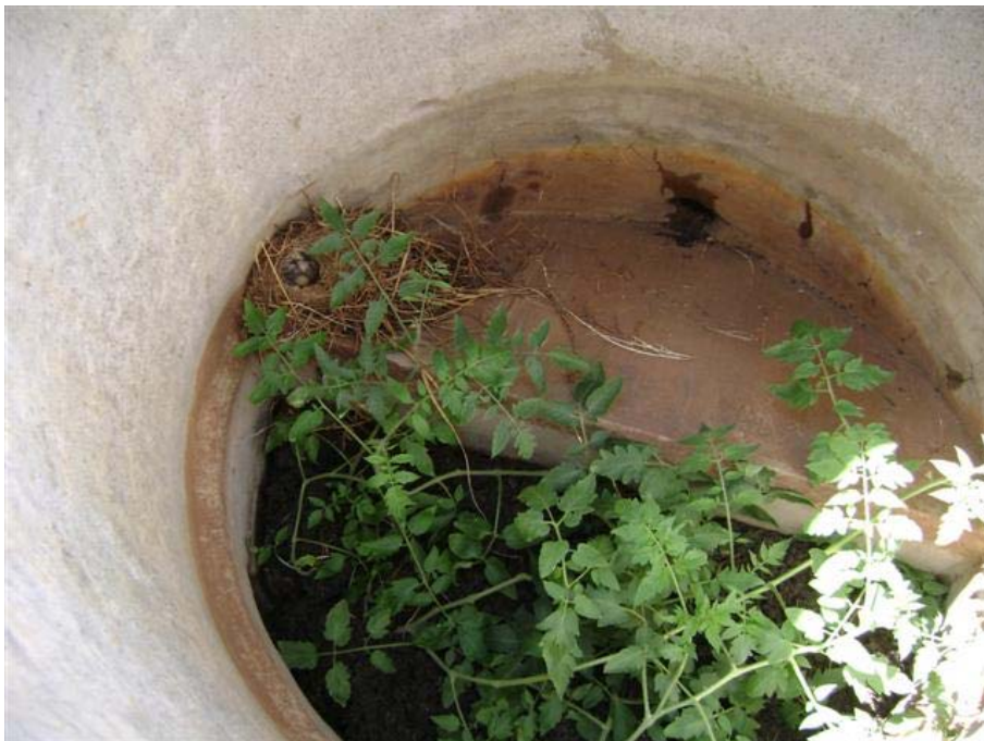
Fig. 80: Sludge storage area inlet chamber, clearly not been used for some months.
