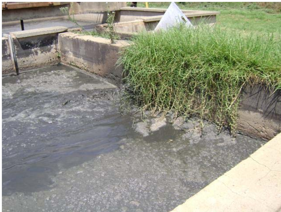
Fig. 70: Poor condition of BNR inlet zones.
