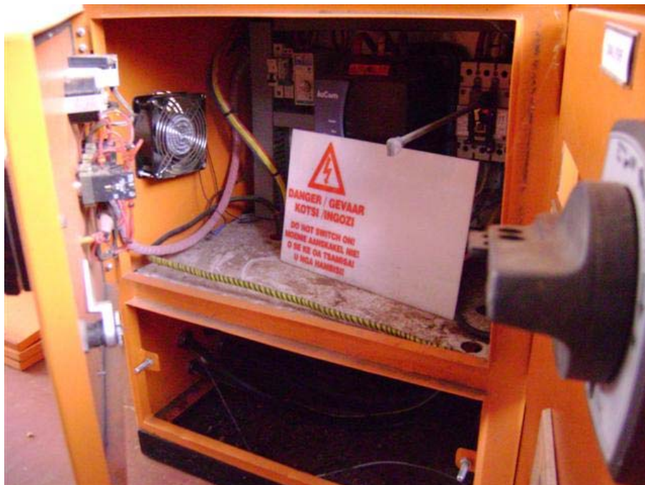
Fig. 86: Inadequate warning or protection against electric shock.
