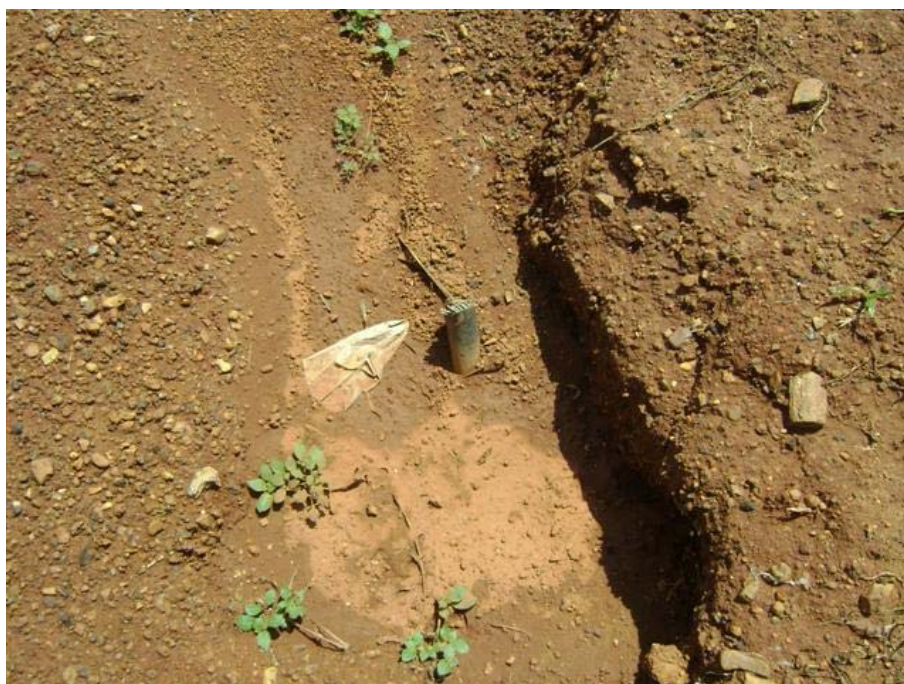
Fig. 87: Electric cable cut off and not protected in any way.
