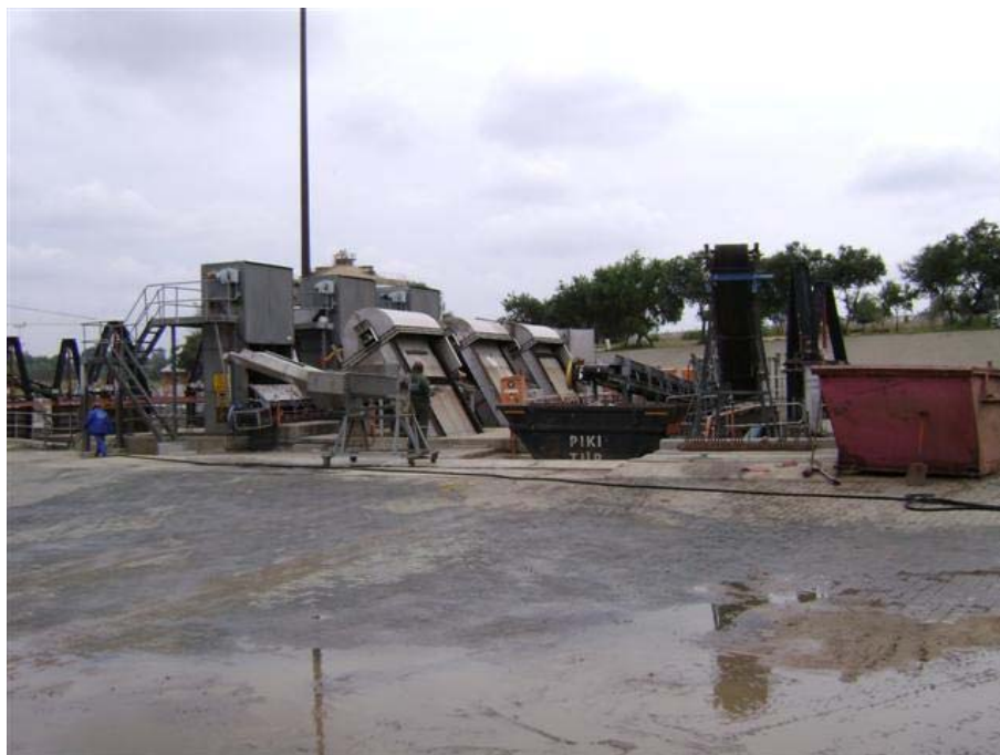
Fig. 43: Grit and screenings properly collected in skips prior to off site disposal.
