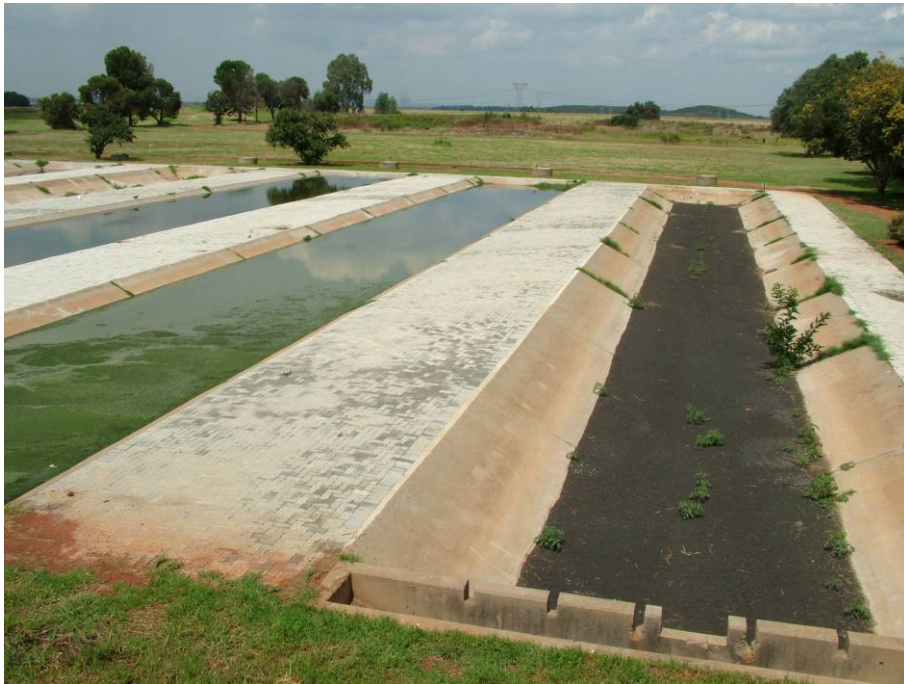
Fig. 79: Sludge drying beds with vegetative growth and algae on surface.
