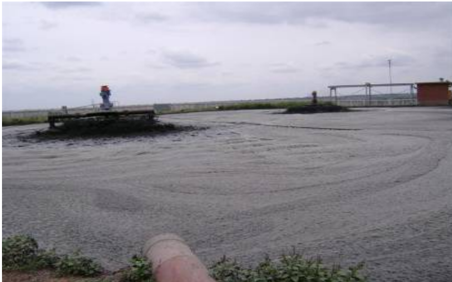
Fig. 27: Sludge holding dam, with floating aerators.
