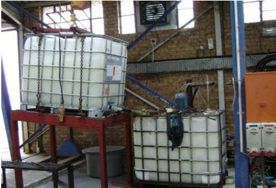
Fig. 36: Polymer dosing plant in use.
