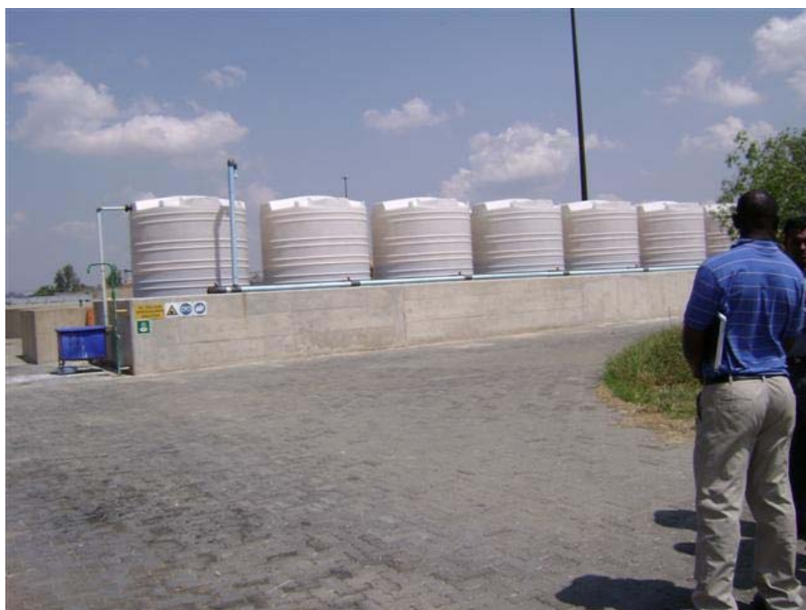
Fig. 57: Hypochlorite disinfection equipment.
