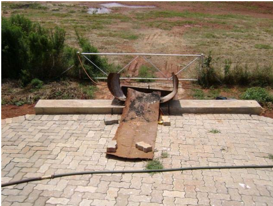
Fig. 64: Unsafe access to skip for rag and grit disposal.
