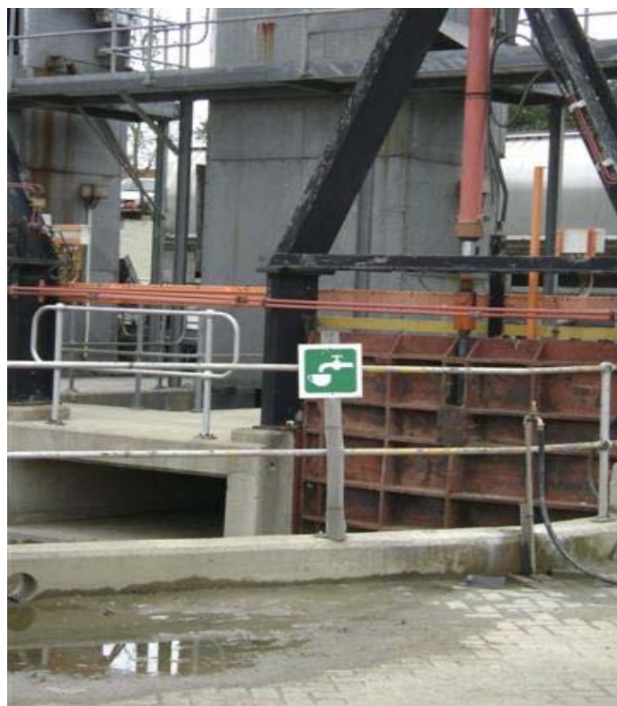
Fig. 58: Drinking water tap – signed, but very close to inlet works channels.
