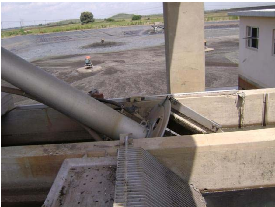
Fig. 62: Mechanical and hand rake screens, also with no fall protection provided.
