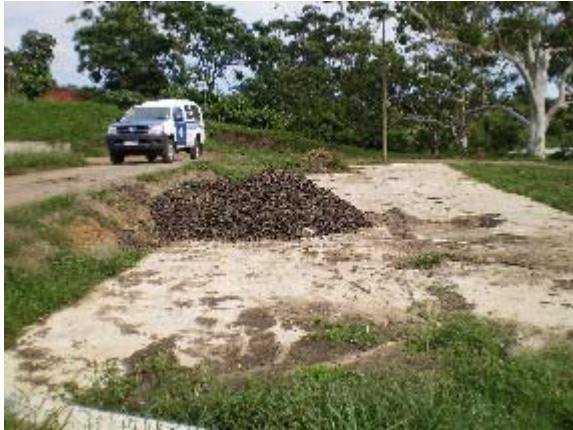
Photograph 1: Dried sludge, stored prior to disposal
