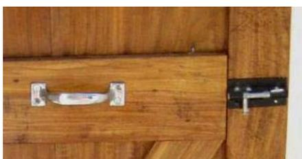
**Figure 4-7: Large internal bolt + handle**
