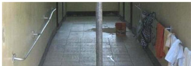
All handrails were circular sections, between 25-75mm diameter and had an average 130mm clearance from the wall. Vertical handrails started 200-470mm from the floor and were 485-600mm in height. Horizontal handrails were fixed between 490-900mm from the floor and were 990-1500mm long (Fig 4-8). Special school toilets had more handrails than toilets of mainstream schools, where not more than one horizontal handrail was ever provided. All handrails were metal,
