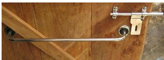
Small padlocks might be difficult for a child to hold and unlock. Fig 4-6 shows a small bolt on the inside of the door and though a handle has been provided to aid door closure, this is also small and would be difficult to reach from a wheelchair. By contrast the internal bolt in Fig 4-7 is easy to grip and the handle of the open door can still be reached by wheelchair users having entered the cubicle.
