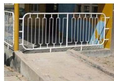
**Figure 4-3: Large steps, drop outside first cubicle**
