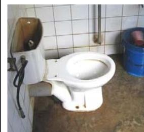
often obstructed access to the latrine (Fig 4-30). Since it is usually considered good practice for taps to be within reach of latrines to allow cleaning before transfer back to a wheelchair, this suggests that greater thought about internal arrangement of cubicles is necessary.
