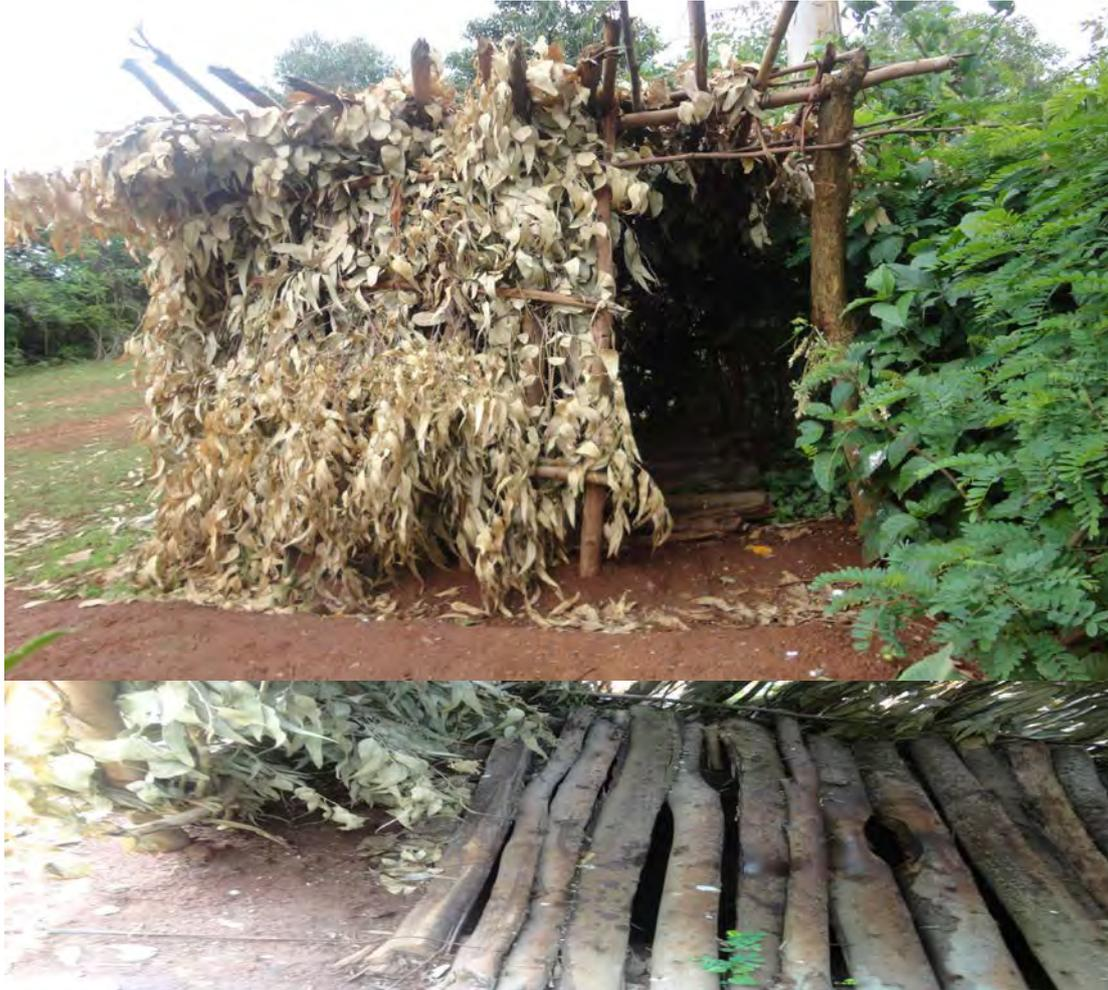
**Figure 4. 3 An example of a road side public latrine with its inside floor of logs**
