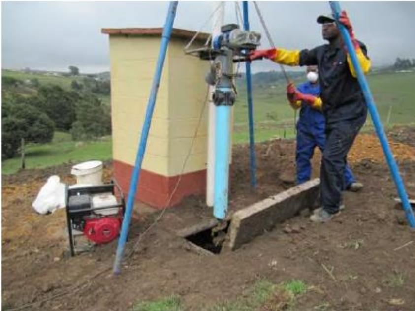
Figure 7 Modified mechanically powered auger (Still & O'Riordan, 2012)
