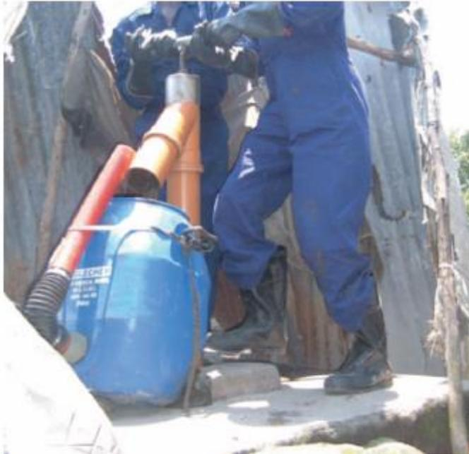
Figure 9 The Gulper emptying FS into a container to be transported (Thye, et al., 2011)
