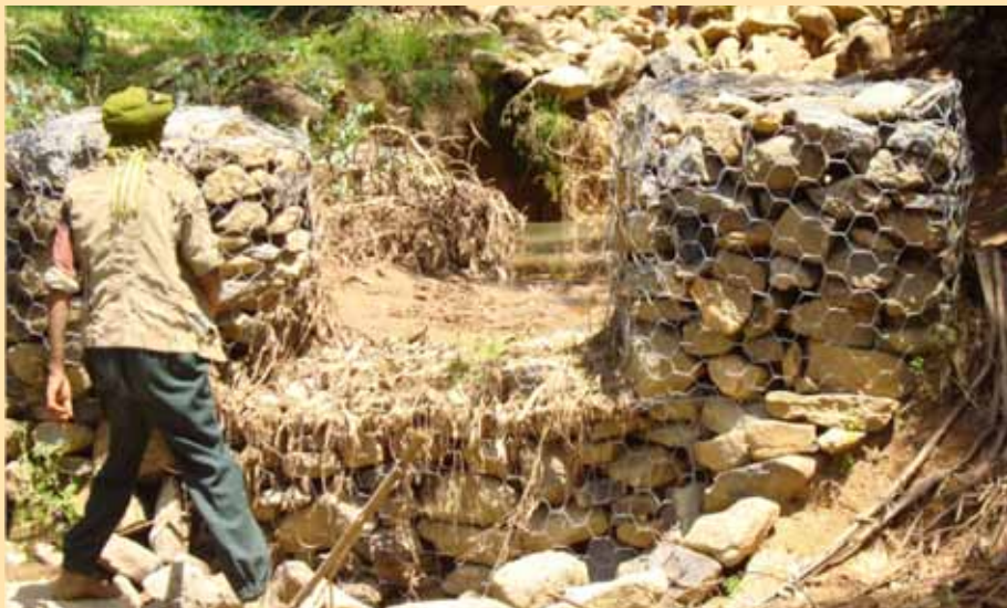
Figure 30. Perfectly functioning gabion checkdam with a spillway and an apron (photo: Lakew Desta)
