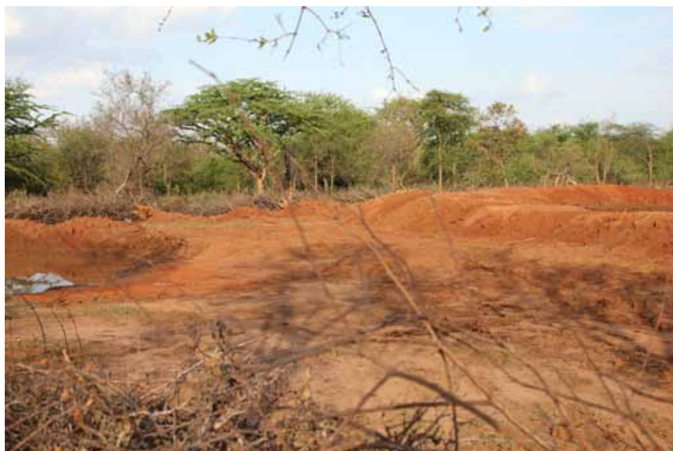
Figure 38. On the right sides of the picture, a part of a trapezoidal bund can be seen. The soil to construct the bund was excavated from the pit on the left side which is also functioning as water harvesting structure (photo: MetaMeta)
