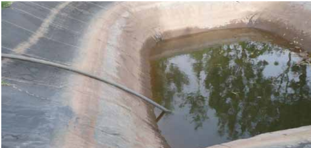
Figure 67. Small lined harvesting pond (photo: Bancy Mati)
