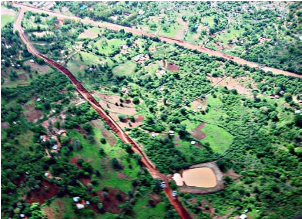
Figure 63. Aerial view of road runoff stored in a hill side dam and used for domestic and livestock water source (photo : Nissen-Petersen)
