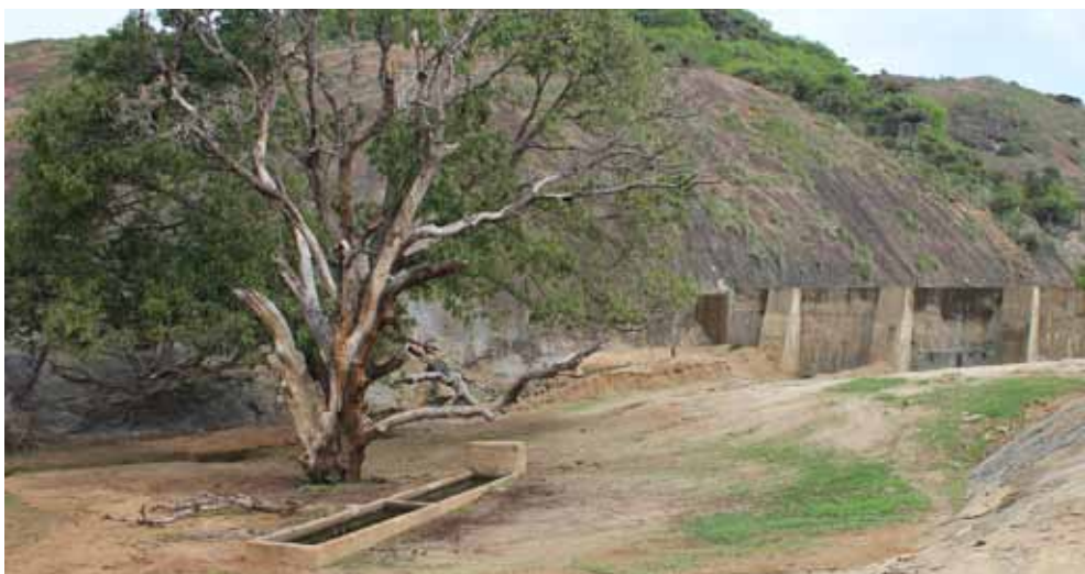
Figure 69. Rockdam with cattle trough (photo: MetaMeta)
