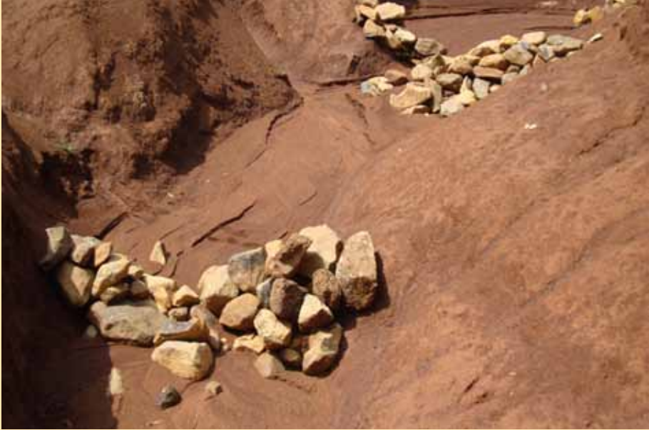
Figure 29. Poor gully treatment. Use of loose stones and undersized check dams are prone to failure (photo: Lakew Desta)
