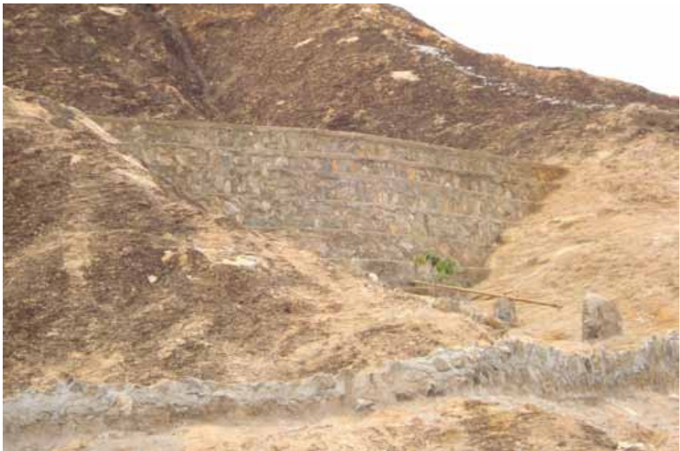
Figure 70. The gutter on the foreground guides the water from the rock catchment to the reservoir. The stone wall is constructed to slow down the speed from the water above preventing the water from overflowing the gutter (photo: WRMA)
