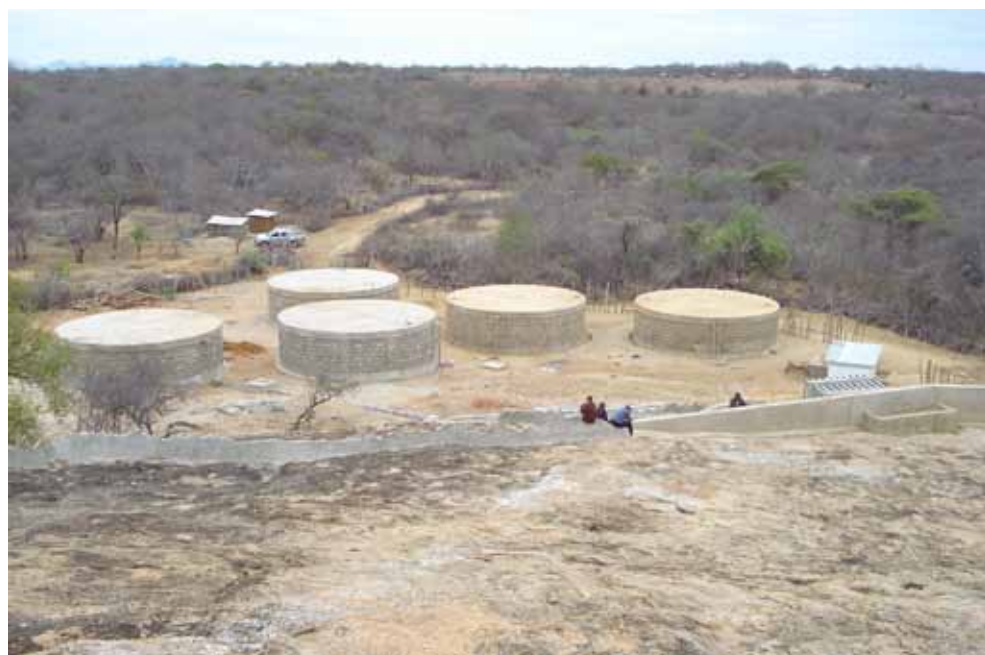
Figure 71. Rock catchment with water tanks (photo: WRMA)
