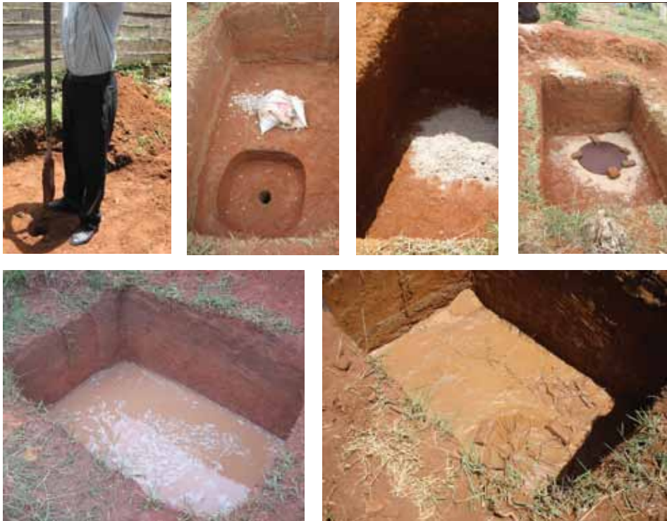
Figure 56. Steps of constructing a tube recharge (photo: Henk Holtslag, Connect International)
