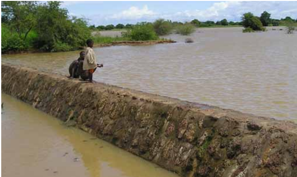
Figure 76. Water spreading weir (photo: GIZ)
