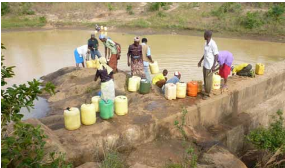
Figure 65. Small dam in a slopy area (photo: Mathias Gurtner, GIZ)
