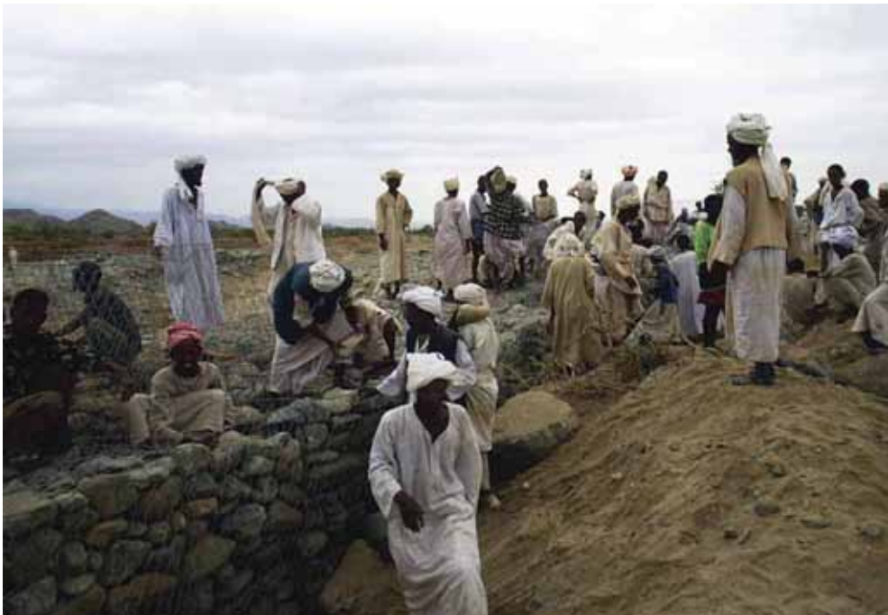
Figure 74. Constructing bunds for spate irrigation (Photo credit: MetaMeta)
