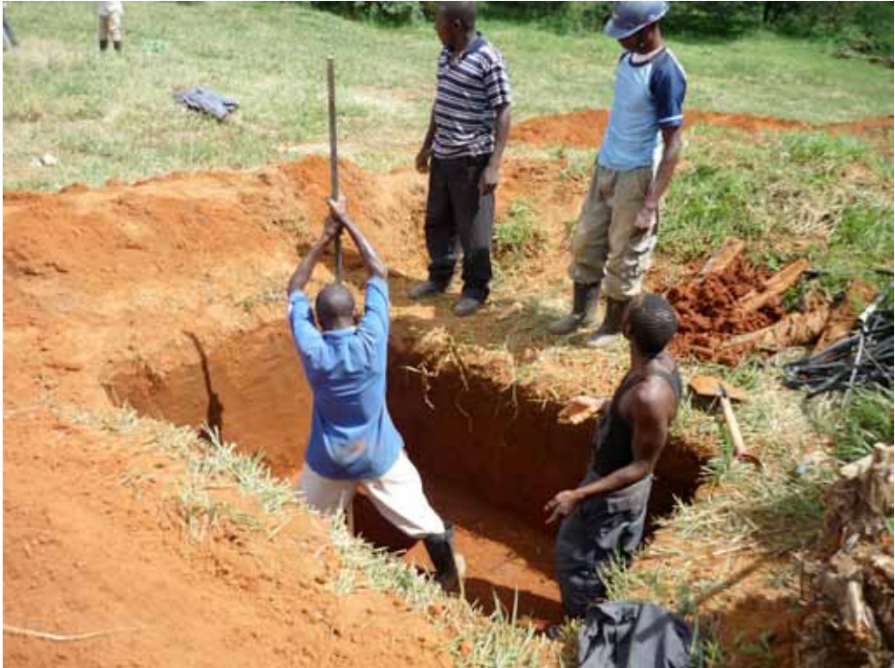
Figure 55. Constructing a tube recharge (Photo: Henk Holtslag, Connect International)
