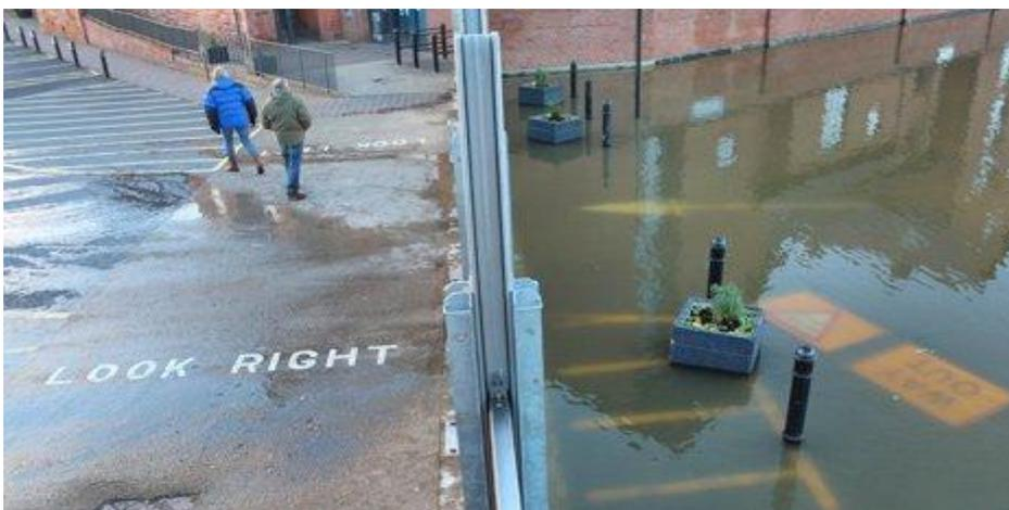
Figure 5.15. Demountable flood defences in Frankwell, Shrewsbury. Source: BBC Shropshire, 2013.
