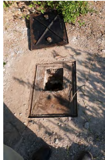
Access cover of ST7:
