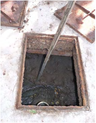
Inspection of ST6:
