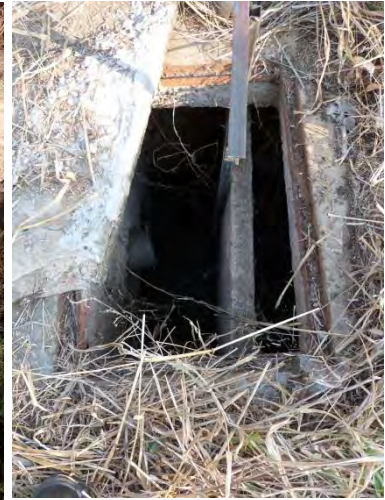
Inlet and baffle wall of ST12:
