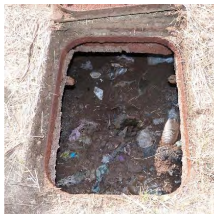
Figure 5.3 – Solidified sludge of ST5. © Mirco Keller.
