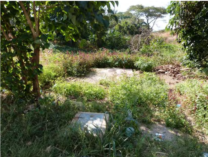
Manhole cover and ST7:
