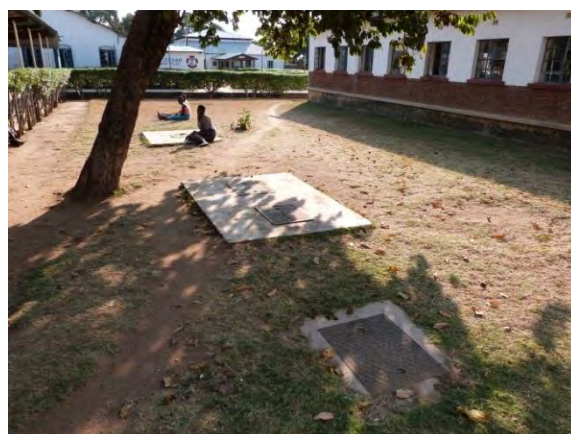
Figure 5.2 – Septic tank (ST6) with soak pit in the background. © Mirco Keller.
