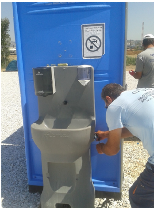
FIGURE 24: WASH STATION ATTACHED TO ROW OF CHEMICAL TOILETS, SOFTEX CAMP (T McMANMON)
