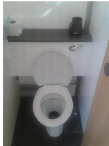
FIGURE 20: RECIRCULATING CHEMICAL TOILET, 'POSH LOO' TRAILER, SIDMOUTH (T McMANMON)
