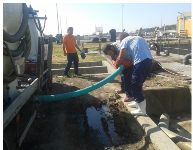
FIGURE 25: DESLUDGING AT WASTEWATER TREATMENT PLANT, SINDOS, THESSALONIKI (T McMANMON)
