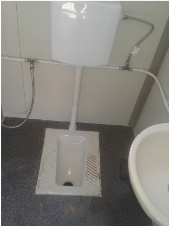
FIGURE 26: UNHCR / IRC CONTAINER CUBICLE SHOWING REVERSED SQUAT PLATE (T McMANMON)
